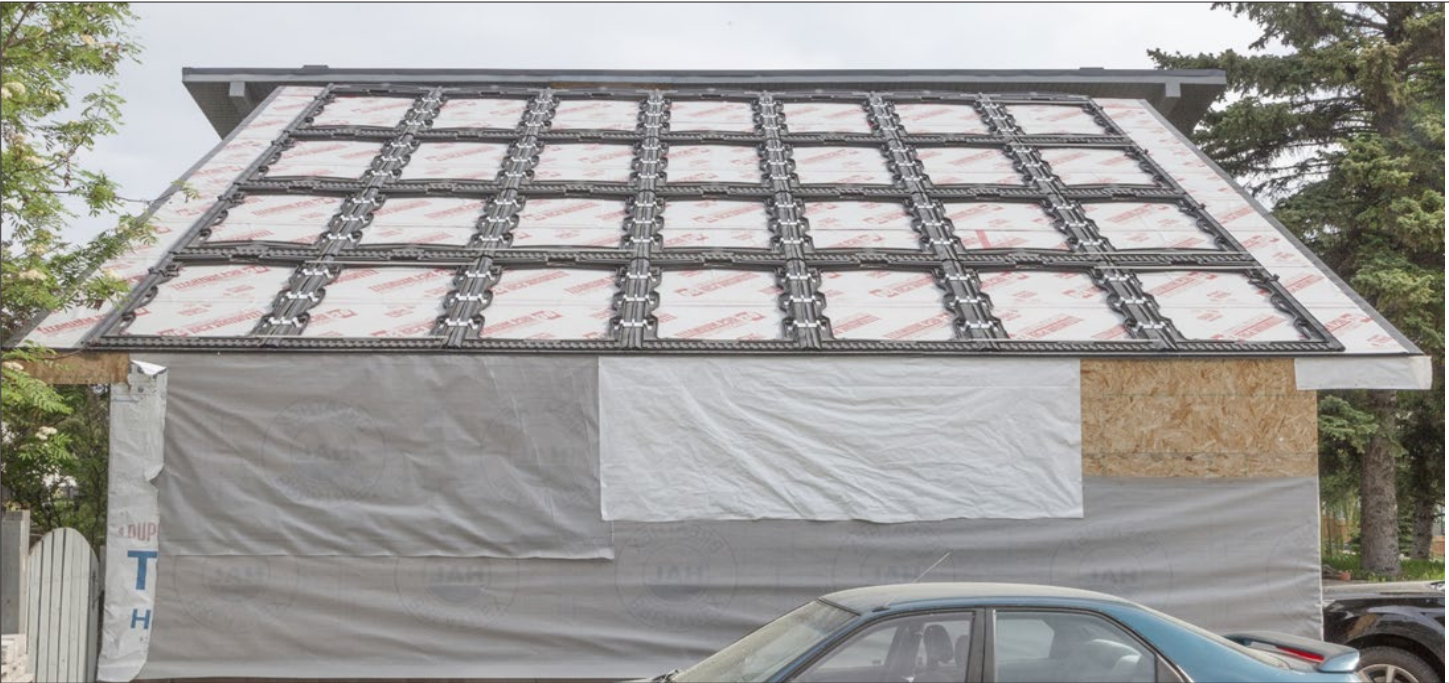
Adjustable frames that can accommodate different PV-panel sizes.
